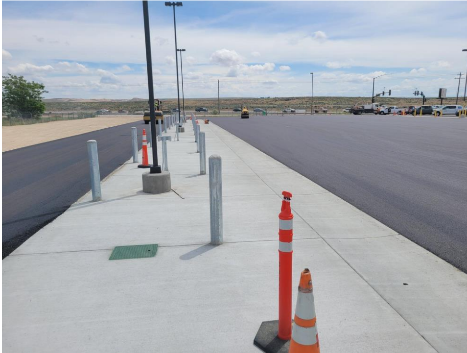
Figure 1: Paving Progress at Orchard
